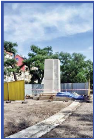
Path for Walk of Freedom with Completed Base and Pedestal
