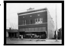
Historic Kosek Building
